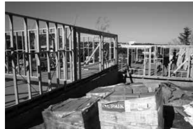
Construction of home for homeless youth
