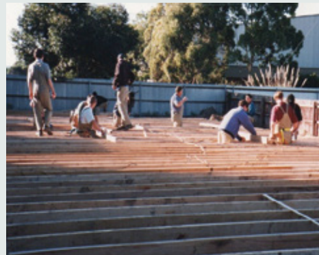
Holmesglen Construction students Children’s Centre construction – Stage 1
